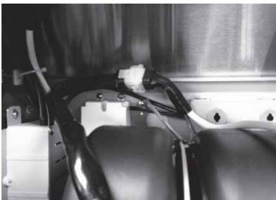
5. Connect 9 pin molex connector from internal motor to 9 pin molex connector from capacitor box cable. Secure cable to hood interior with zip tie and zip tie holder.
