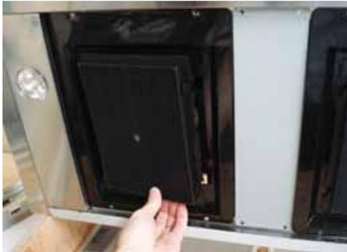
3. Install charcoal filters into charcoal filter brackets
