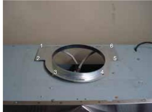
2. Secure 7" round collar to top of hood using (6) M4 x 6 screws.
