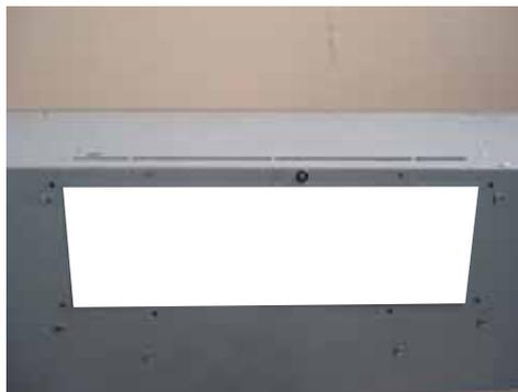
1. Using a flat-head screwdriver, remove the rectangular knock-out plate located on back of hood.
