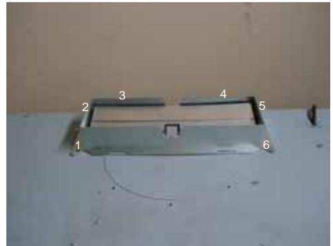
2. Secure 3-1/4" x 10" rectangular collar to top of hood using (6) M4 x 6 screws.
