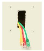
**Fig.8:** The three Cat-5e cables have been installed and pulled through the rectangular opening in the wall.
