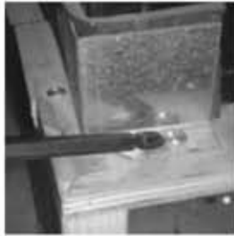
Image 1 Removing bracket from skid
