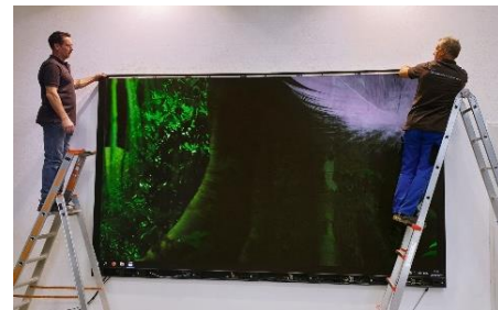
Figure 60: Installing Overframe (top)
