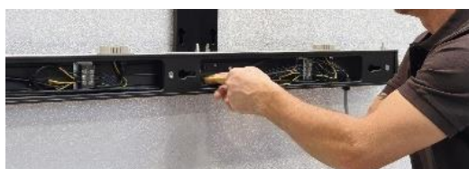
Figure 45: Wall Mounting: Attachment of Power Bar (Detail)
