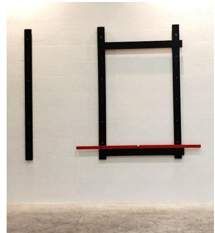
Figure 43: Using Alignment Bar with Spirit Level
