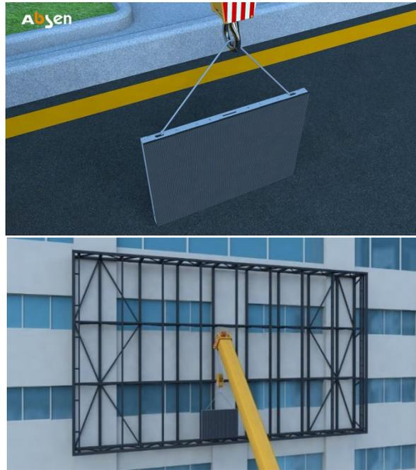
Step 3: Place a second cabinet on the left or right side of the first cabinet. Put them next to each other. Use a wrench to lock the M10 bolt into the mounting hole of the cabinet. , Then use bolts and screws to lock the two adjacent cabinets tightly
