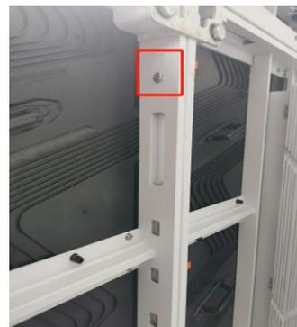
Step 4: Follow the previous steps to install the third cabinet, the fourth cabinet...until the installation of the first layer of cabinet is completed.
