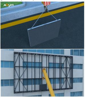
Step 3: Place a second cabinet on the left or right side of the first cabinet. Put them next to each other. Use a wrench to lock the M10 bolt into the mounting hole of the cabinet., Then use bolts and screws to lock the two adjacent cabinets tightly
