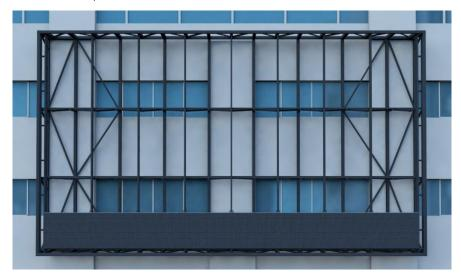
Step 5: Then install the second layer of cabinets. First, place the cabinets in the middle of the second row, adjust the horizontal and vertical flatness, and then use bolts to lock them tight.
