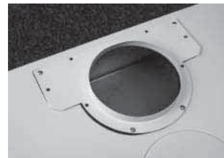
2. Remove top pre-mounted transition piece.
