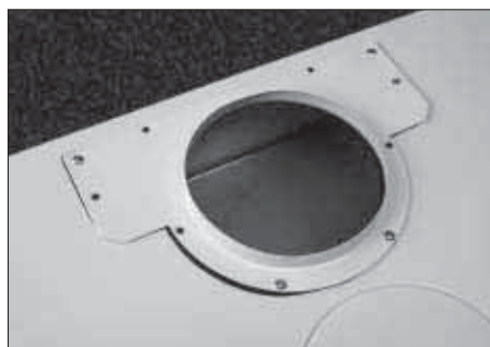
1. Remove pre-mounted 6" transition adapter or duct opening.
