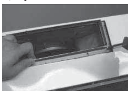
6. Mount starting collar (provided) at rear discharge.
