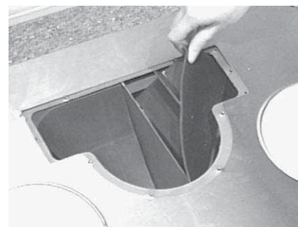
3. Remove 2 air diverter blocks through top opening as shown.
