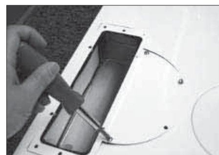
4. Mount rectangular transition piece to top opening as shown.
